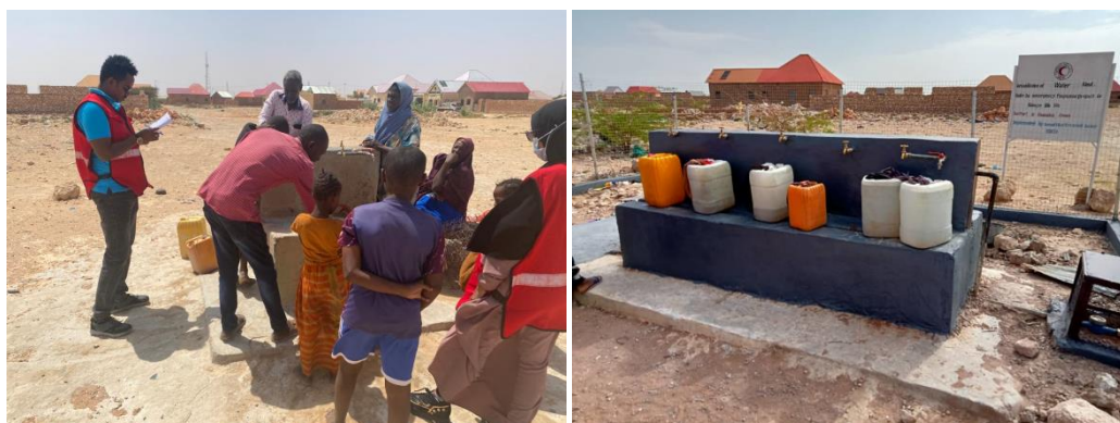
Water collection points before and after the rehabilitation
